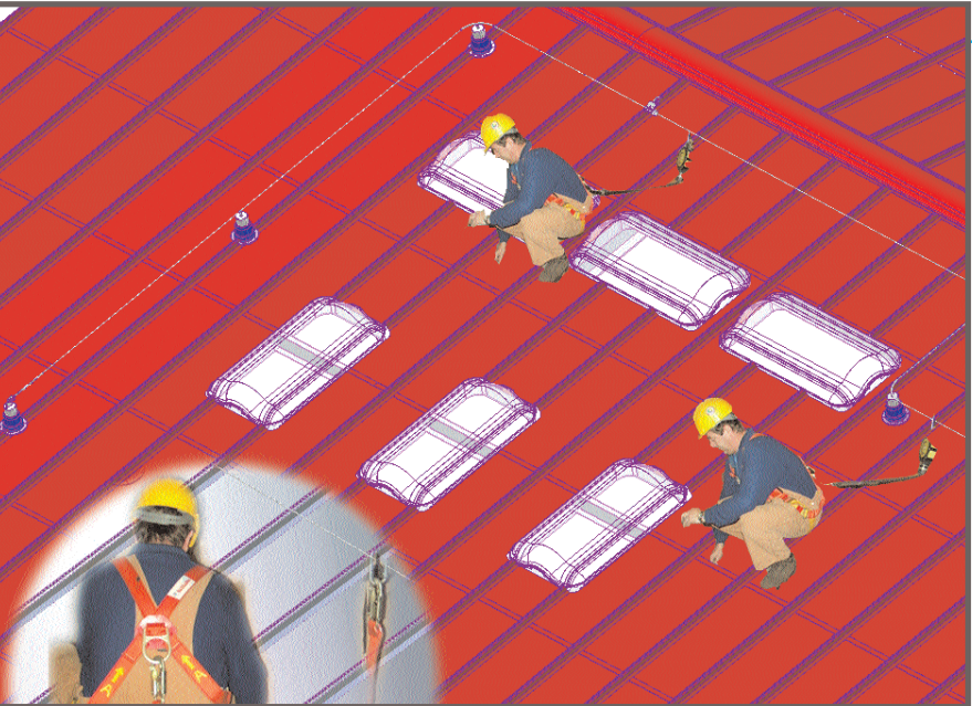
Maintenance Personnel Working Around Skylights, A Recognized Fall Hazard Area (Brittle Skylight Problem)
